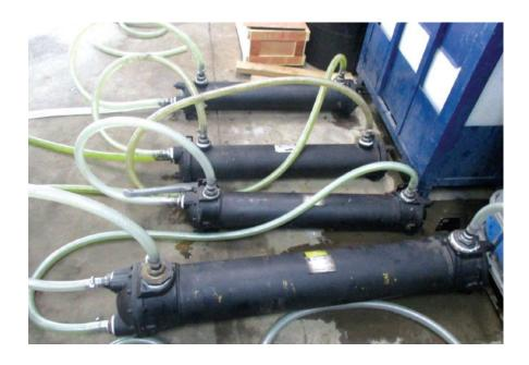
\*The level of success for this cleaning method is determined by the amount and type of contamination. If the scale has hardened, which is very common on heating applications, the chemical flush effectiveness can be limited.
