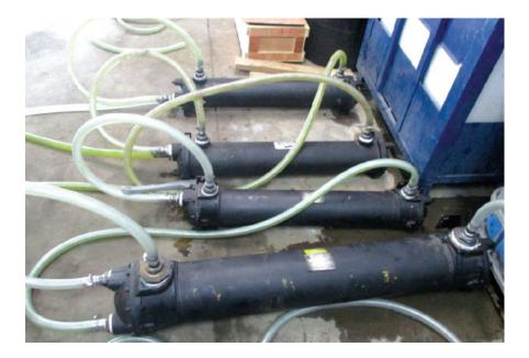
\*The level of success for this cleaning method is determined by the amount and type of contamination. If the scale has hardened, which is very common on heating applications, the chemical flush effectiveness can be limited.
