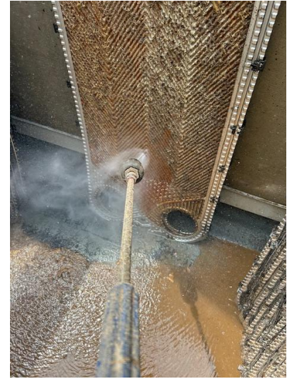
3500 PSI Water c/w Rotary Nozzle
