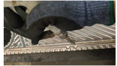
Applying 3M #1099 Rubber Adhesive
